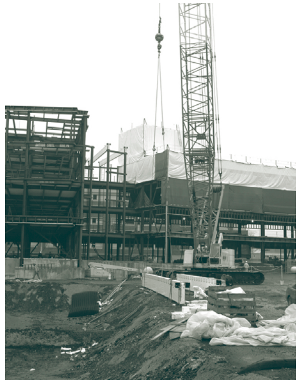
The third beam is readied for placement.
