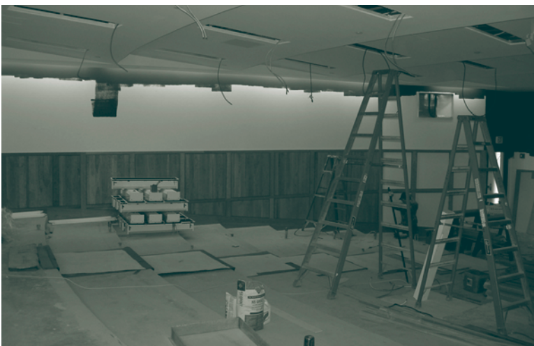
Steimer Auditorium under construction, January 2006.
