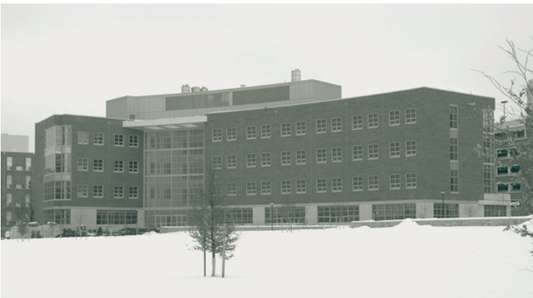
Forest Resources Building, Park Avenue view, December 2005.
