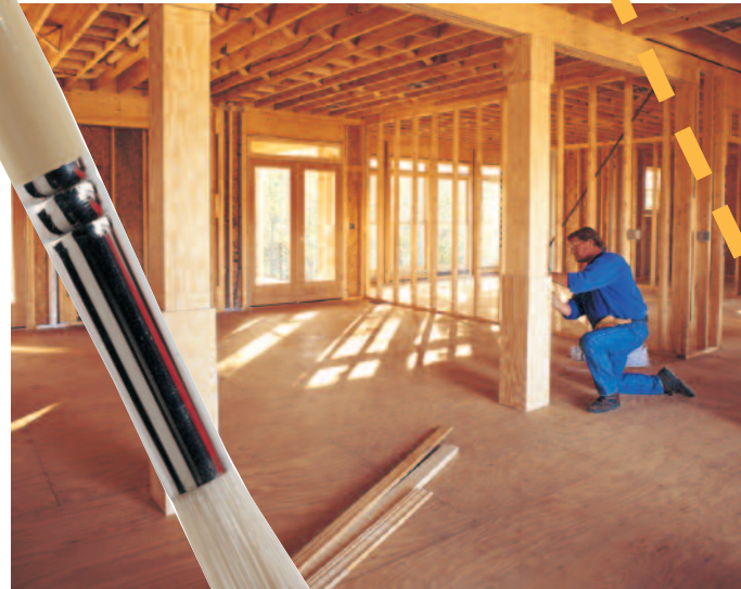
NEW HOME CONSTRUCTION
