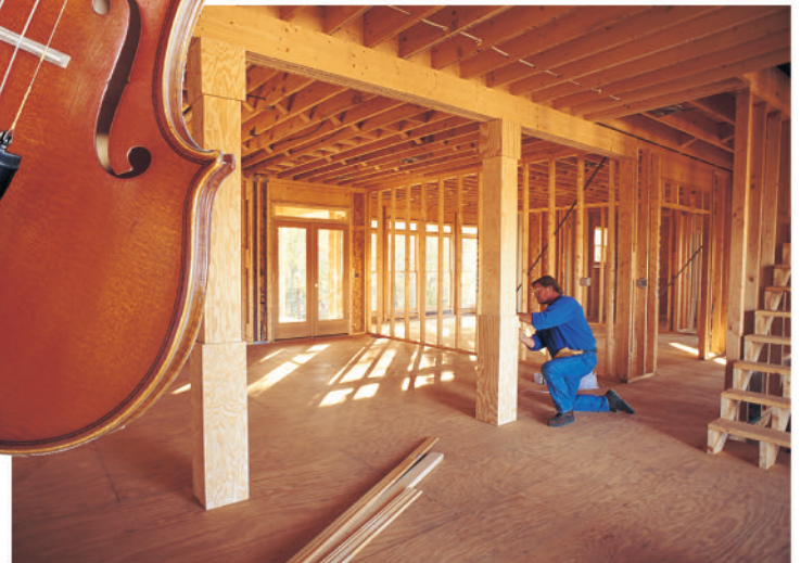
NEW HOME CONSTRUCTION
