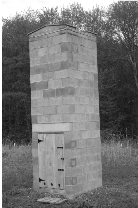
The completed Chimney Swift tower is ready to welcome its first pair of inhabitants.
