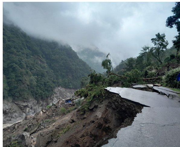
Fig 3b. Road connectivity severely affected at the Rithcu Village in North Sikkim. Courtesy: Dupjang Lepcha, ATREE
