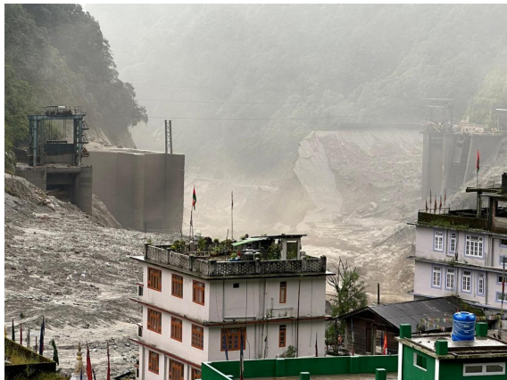
Fig. 7a. The destroyed Teesta Stage III dam at Chungthang. Courtesy: Anonymous
