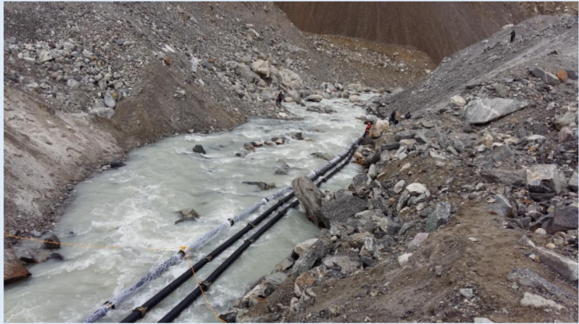
Fig 5. Siphoning water to reduce the lake levels at the South Lhonak Lake. Courtesy: Sikkim Government Technical Report
