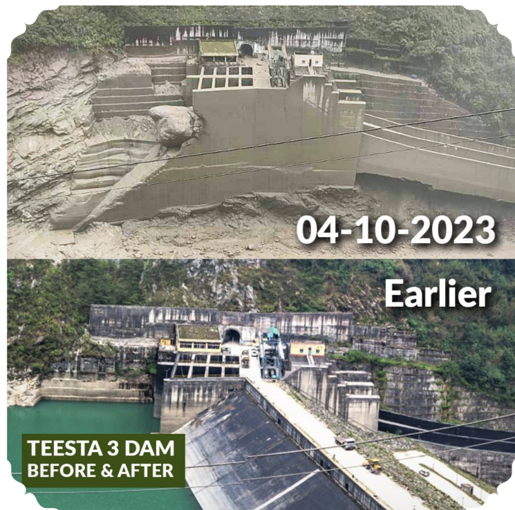
Fig. 1. Teesta III Hydropower Plant, Sikkim, before and after the Oct. 4, 2023 flood. Credit: https://sandrp.in/tag/teesta/
