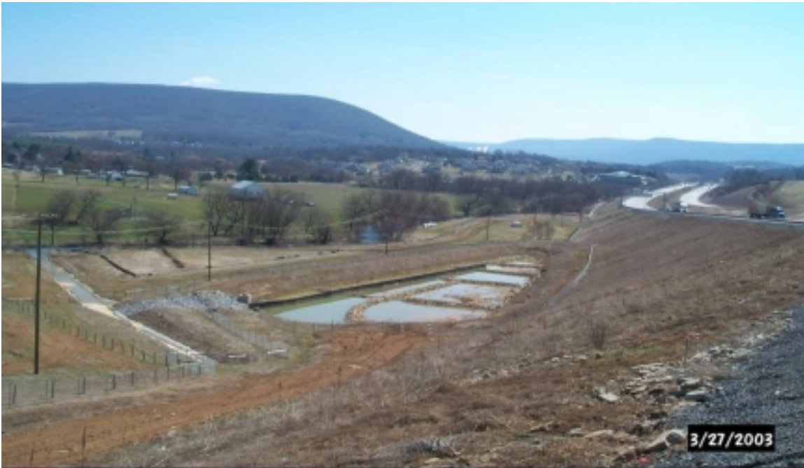
Picture 4. An overlook of the Park Avenue site from the Rt. 322 exit to the new highway at the completion of construction activities. A stormwater detention basin is in the middle of the picture and concrete drainage channel is to the left.
