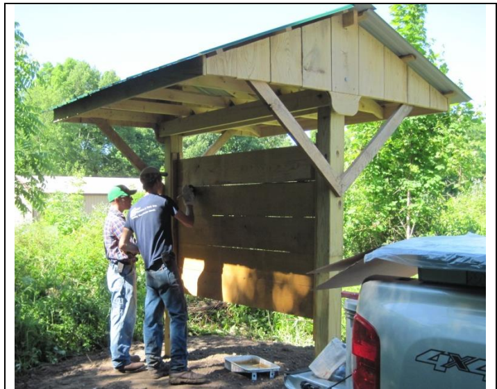
Nicholas Heban and Charley McCaw applying “Cabot” stain to the horizontal ash boards. (Note the diagonal bracing)
